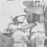
THREE READ-Mix trucks kept concrete hoppers, above, continually filled in the dawn to dusk operation. After a two-cubic-yard hopper, left, was filled, it was swung out to the dolphin by Raymond's big crane, lower left, and dumped in the steel reinforced base, lower right.
